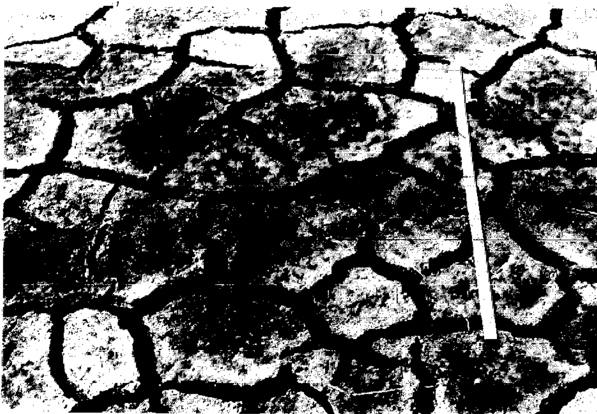
Fig 4. Pond bottom is sun-dried till it cracks
