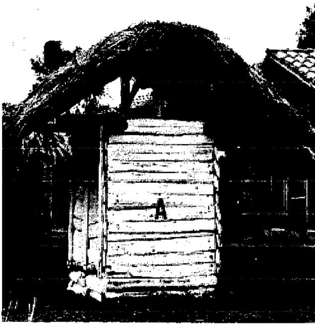
Figure 21. Simple, small rustic stores with outside painted white. A -- Timber construction, 1.5 TM capacity (CIP, Huancayo, Peru). B -- Lath and plaster and mud brick construction, 2 TM capacity (Mountain State Agricultural College, Baguio, Philippines).
