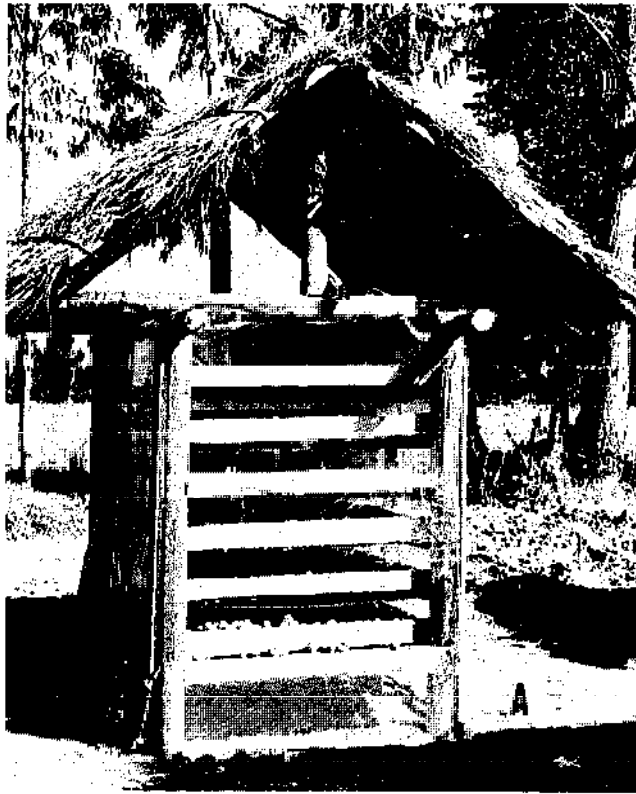
Figure 31. Small-scale natural diffused light stores using fixed shelves and local building design and materials. A - CIP, Huancayo, Peru. B - Sayangan, Philippines. C - Nigale, Nepal.
