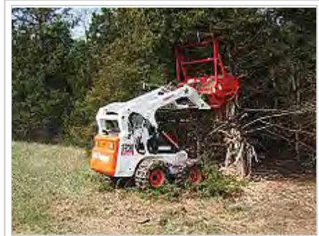
Forestry mulching attachment on a Bobcat skid steer
