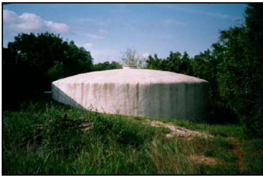
Figure 2-10. Ferrocement tanks, such as this one, are built in place using a metal armature and a sprayed-on cement.
