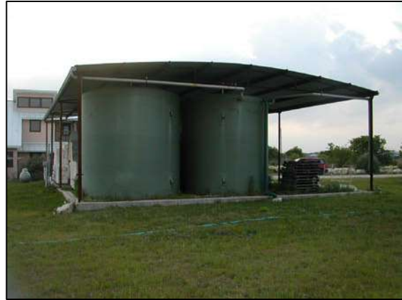
Two 10,000-gallon cisterns collect rainwater at the Pomerening/Dunford residence in Bexar County.
