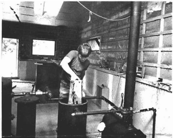
Fuel being added to combustion chamber.
