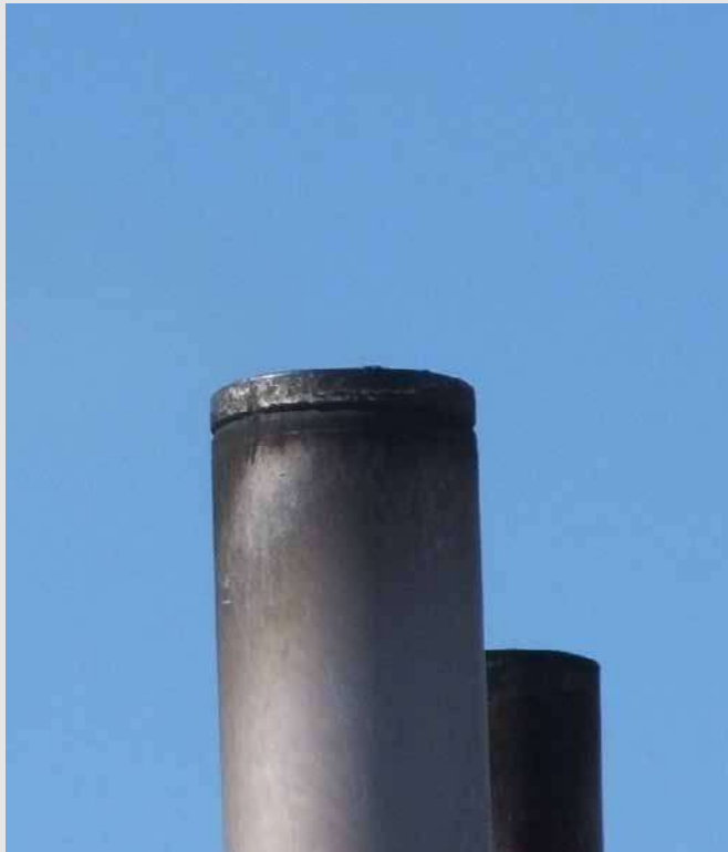
Twelve minutes after start up. ... Still some slight smoke. Camera didn't pick it up.
