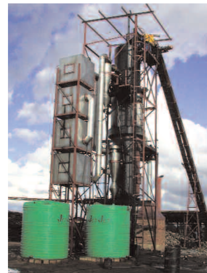
Figure 2: RWC's Slow Pyrolysis facility
