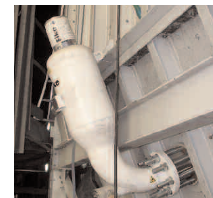
Figure 4 a & b: Anti-explosion bottles for protecting the fuel bins and pipes conveying air and wood dust mixtures.
