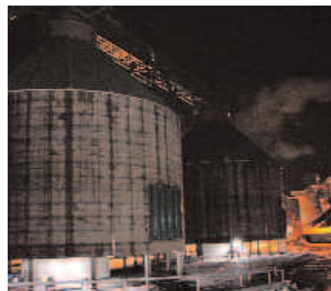
Figure 2: Outside view of the Timelkam plant with fuel bunkers.
