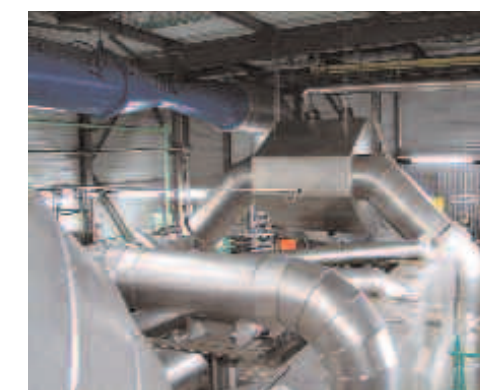
Figure 3: View of the boiler top
