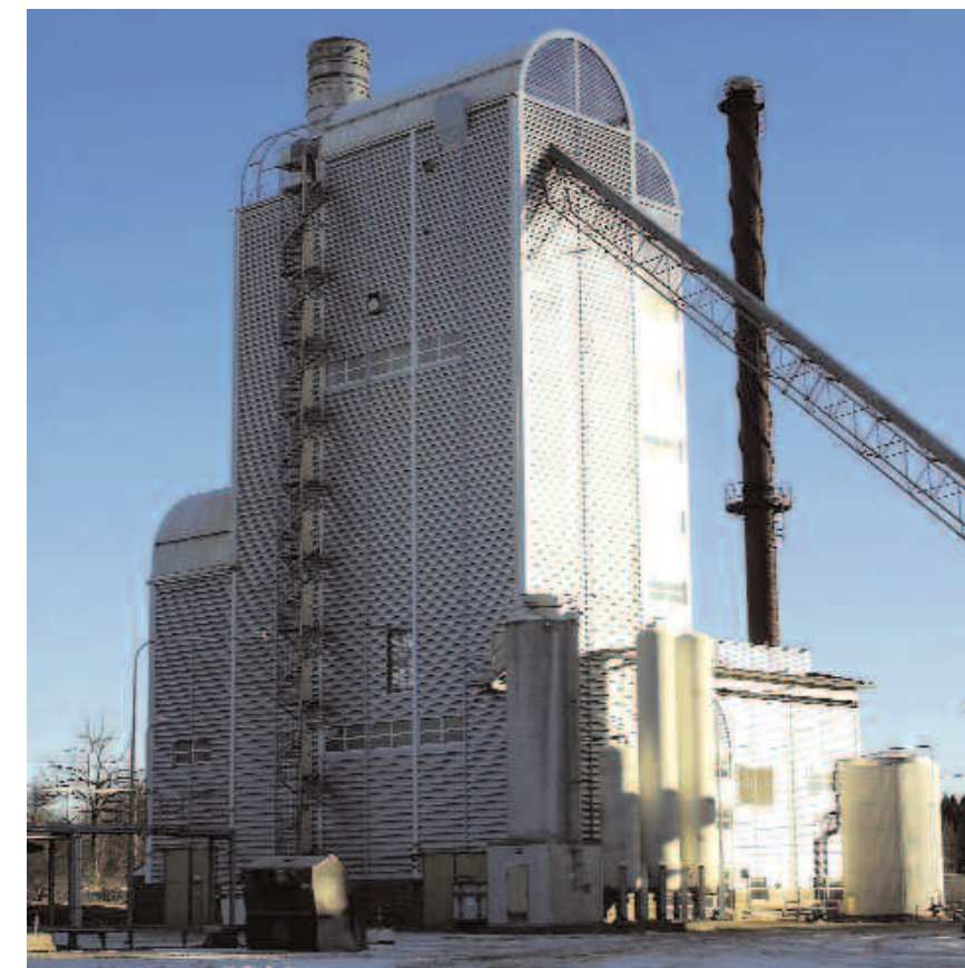
Figure 1: The Värnamo Plant, Sweden.
