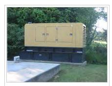
A 200 kW Caterpillar diesel generator set in a sound attenuated enclosure used as emergency backup at a sewage treatment substation in Atlanta, United States.
