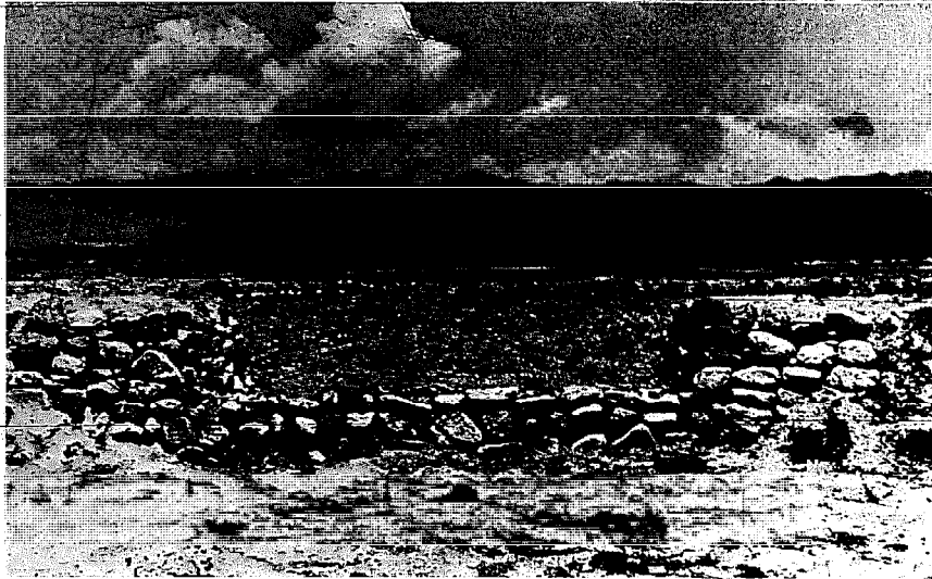
Afghanistan: Spillway made of piled-up stones. The remaining part of the dams is made of earth.
