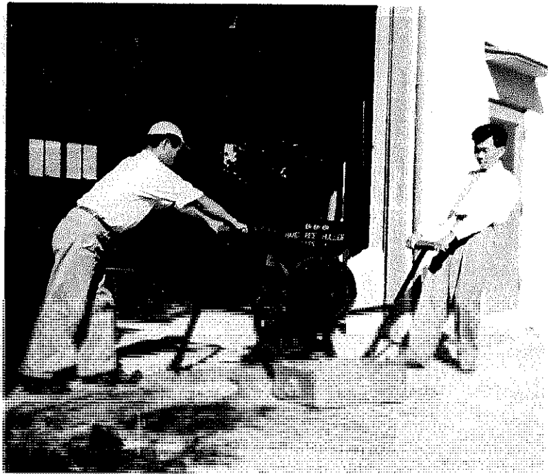
"CECOCO" TWO-MAN HAND RICE HULLER
