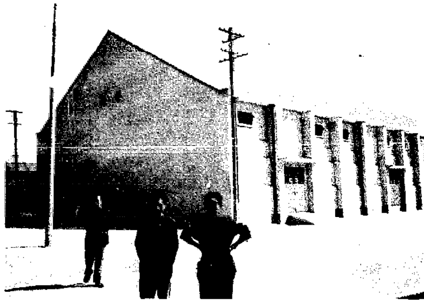
Photo 44 - Type "54" bulk grain warehouse, 20 x 52 m. (First Depot, Wuxi)
