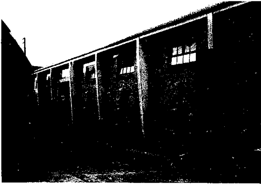
Photo 49 - Warehouse for bagged grain. Portal frames at ca 4 m. Buttresses between portal frames. (Seventh Depot, Shanghai)
