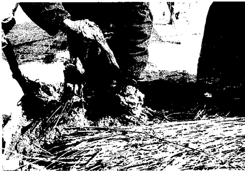
Photo 25 - When straw bundles are thoroughly covered with clay mud, excess mud is removed. (Niou Pao Tin Depot)
