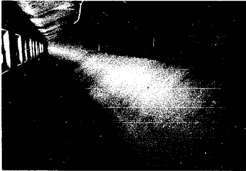
Photo 41 - Type "51" bulk grain warehouse. Wooden building frame and ceiling. Pile height 3 m at wall and 5 m at centre for paddy. (First Depot, Wuxi)
