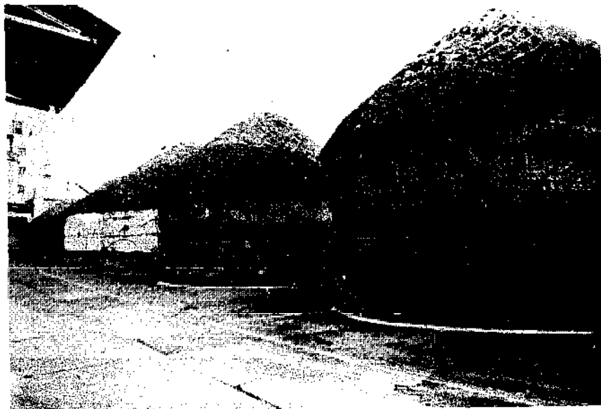
Photo 63 - Outdoor bulk storage for 150 tons of paddy. Walls built from bags filled with paddy, interior space filled with bulk paddy. The top cone is shaped by straw piled on top of the rice, then thatched and fixed with a rope net. (Xinqiao Grain Purchasing and Supply Station, Songjiang County)
