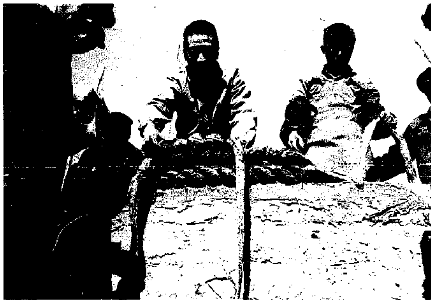
Photo 33 - Third layer of eaves. The top surface must be kept level by placing clay/straw bundles along the wall. (Niou Pao Tun Depot)
