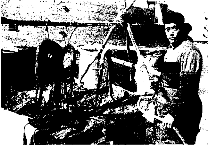
Photo 24 - Mud in half oil drum. Water being added to adjust consistency. Clay/straw bundles hanging above drum. (Niou Pao Tin Depot)
