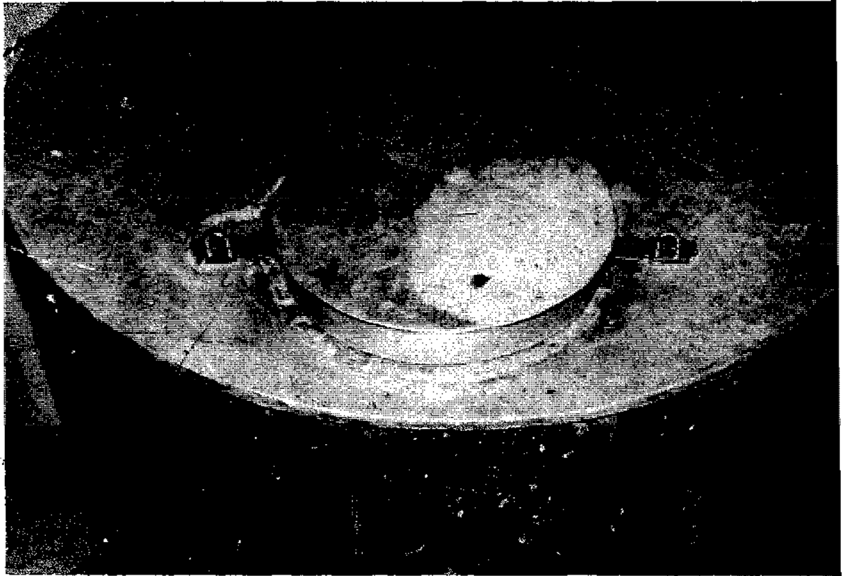
Photo No. 14: Inlet lid with locking arrangement
