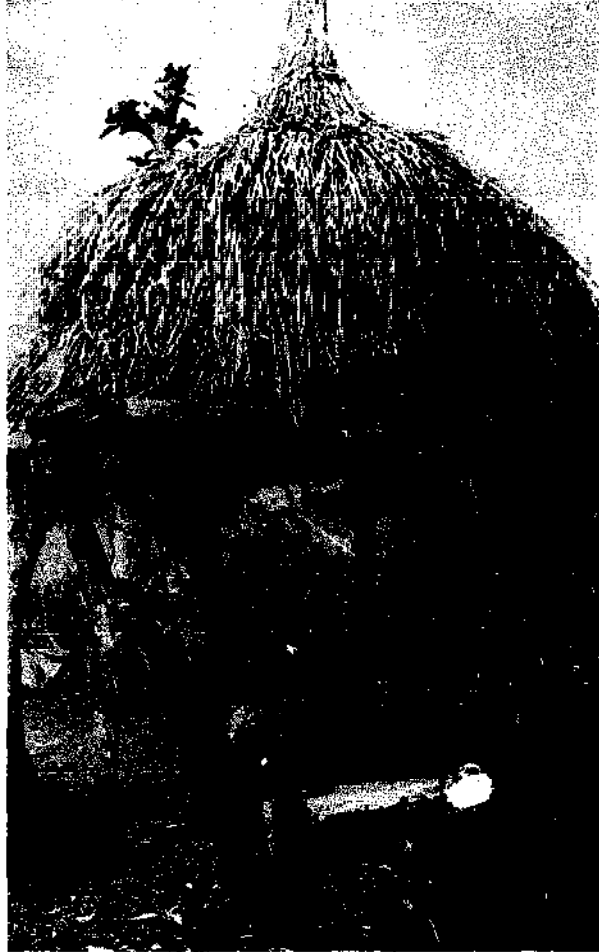
FIGURE 32. Food grains dried on a timber and grass platform over a fire, and covered by a thatched roof.
