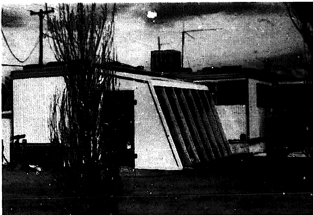
Greenhouse on Mobile Home. Built in Workshop by Mojave County Solar Energy Commission: Kingman, Arizona
