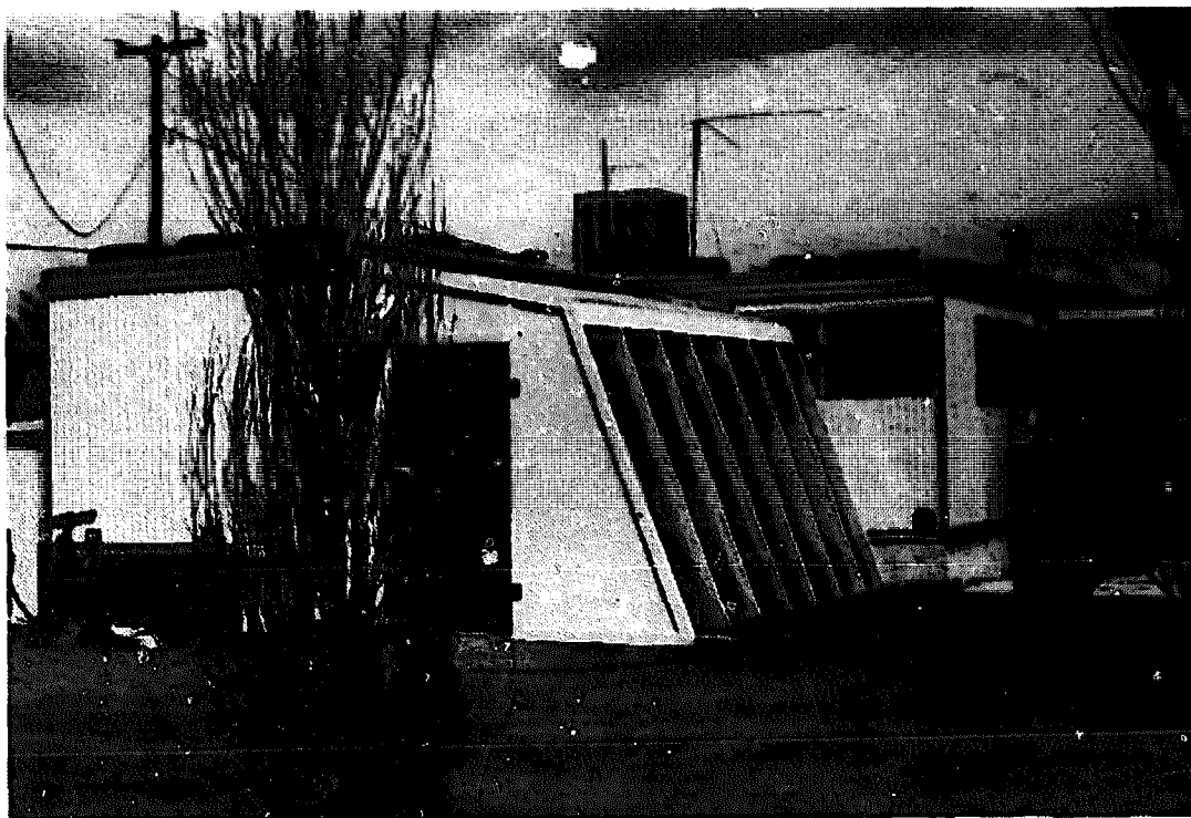
Greenhouse on Mobile Home. Built in Workshop by Mojave County Solar Energy Commission: Kingman, Arizona
