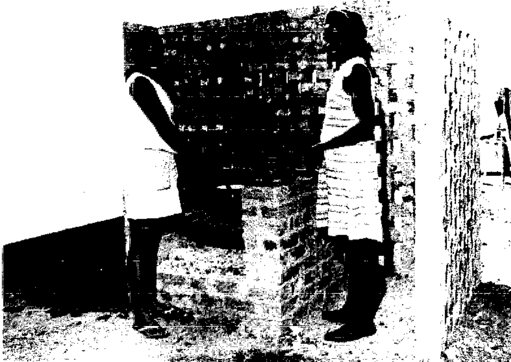
Figure 6.10 Open air oven and charcoal burner used at the Makeni centre
