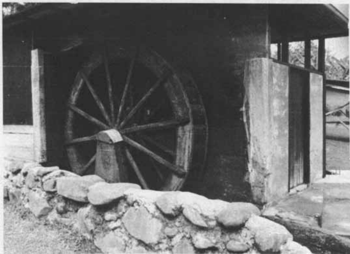
Overshot water wheel (above) and generator (below) at the Swiss Mission near Minj, WHP. Power is transmitted through a counter shaft in order to increase the rpms.
