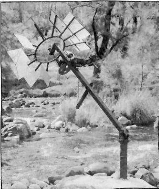
Hoisting the waterwheel out of the river to avoid flood damage.
