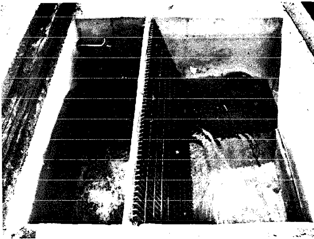
Photo 7 — Inlet arrangement shows overflow pipe and trash rack, top of the pipeline is half submerged on the right hand side
