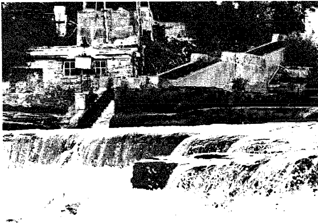
Photo 19 — Waterfall with Denil fish pass
