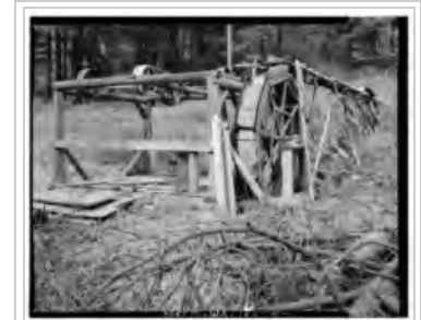
Directly water-powered ore mill, late nineteenth century
