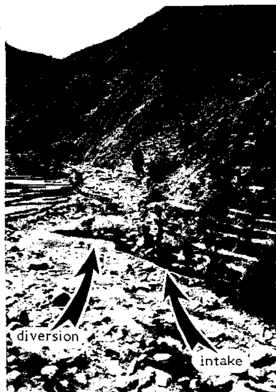
Fig. 4. A temporary structure across the river diverts a portion of the water into an irrigation canal at the right. Similar structures are used with hydropower schemes.
