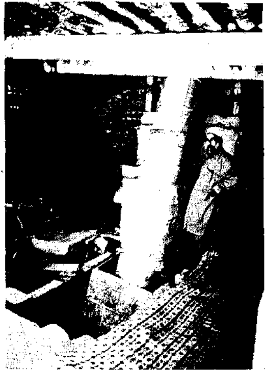
Fig. 17. Oil drum penstock at the Alpuri powerhouse. Operator's bed is in foreground.
