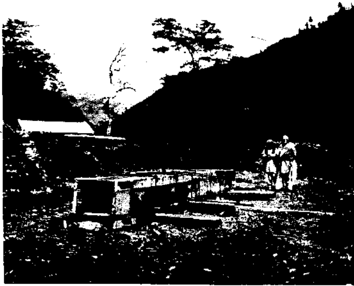
Fig. 15. Wooden penstock for use at the micro-hydro scheme at Mandal.
