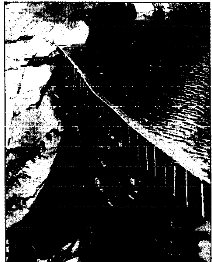
Fig. 5.42. A wooden frame and deck dam.
