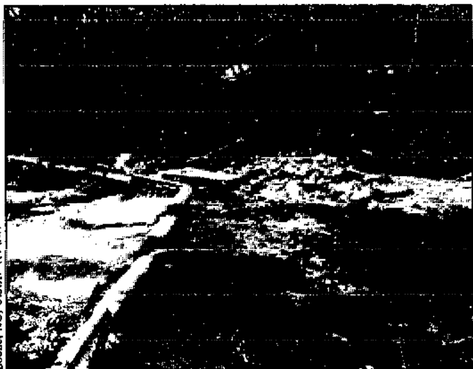
Fig. 5.35. Although this scheme had been shut down for repairs on the penstock, it is apparent that, by crossing the stream obliquely, the weir has caused the stream to transport and drop bed load and sediment directly in front of the intake.
