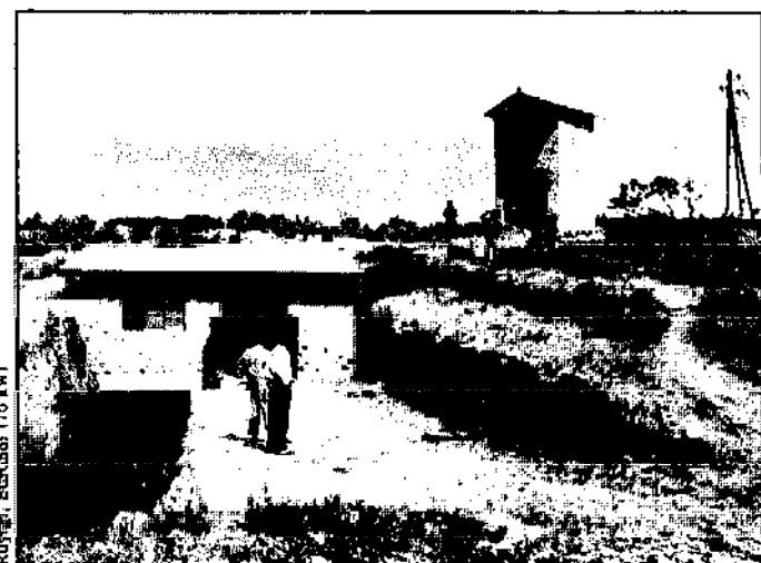
Fig. 4.26. To minimize penstock length, the powerhouse was built in rock below ground level. The forebay is located 10-20 m behind the powerhouse but is not visible. The structure to the right houses an 11 kV transformer.
