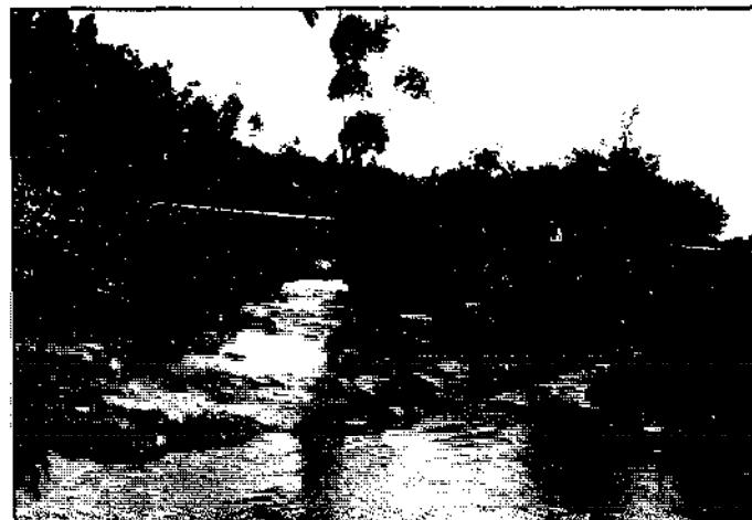
Fig. 5.26. A simple weir of loose stones diverts water to a small turbine-driven mill.
