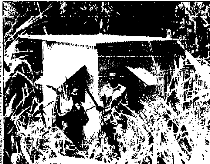
Fig. 5.164. This powerhouse is constructed of flat galvanized steel sheets over a timber frame. Although no permanent windows have been incorporated, shutters constructed in the same manner as the walls can be opened to provide for light and ventilation during visits to the powerhouse.
