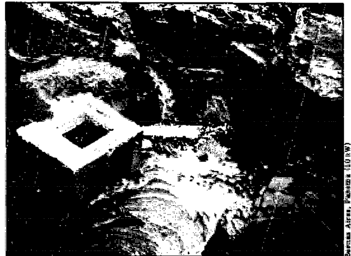
Fig. 5.65. A concrete box behind the small weir serves as the intake. The opening on top of the intake structure is usually closed with a removable concrete plug. A portion of the penstock pipe can be seen between the box and the base of the weir. Several features of this design could have been improved to facilitate maintenance.
