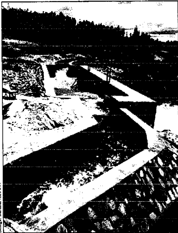
Fig. 5.203. A view of the settling area taken from the dam crest at a site under construction. Two sluice gates permit this area to be scoured out. The sediment returns to the stream at the right.
