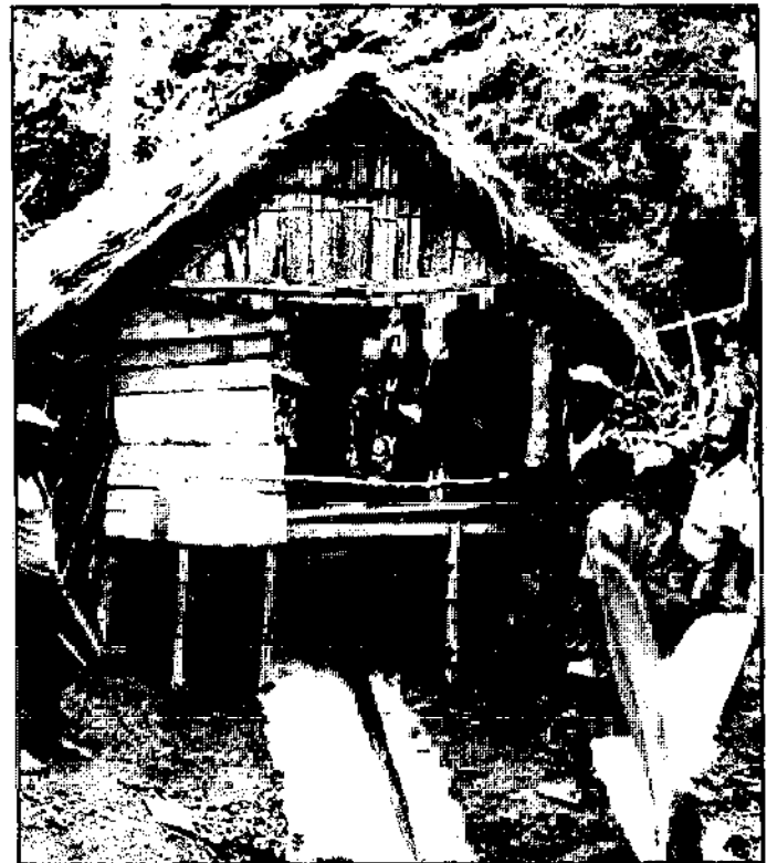
Fig. 5.165. This powerhouse design permits use of indigenous skills and materials—bamboo and thatch.
