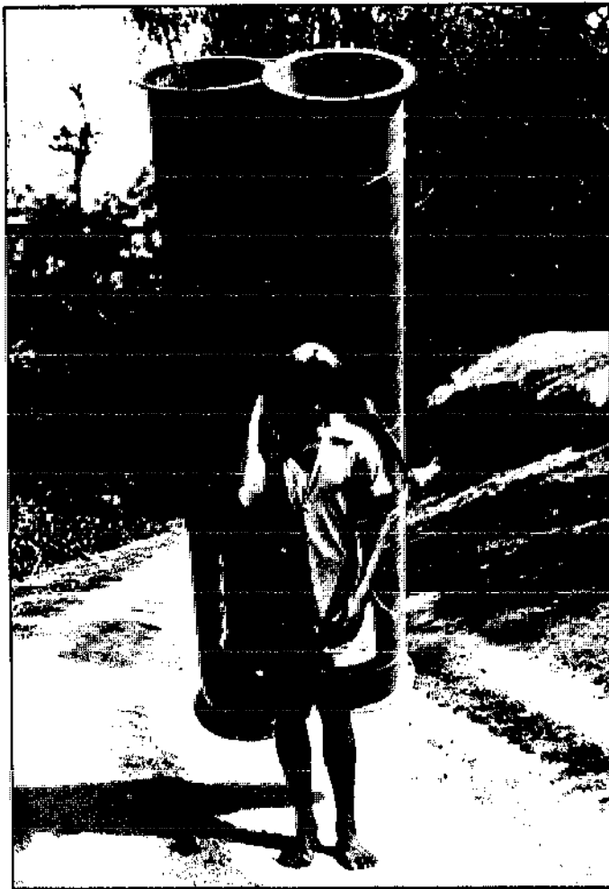
Fig. 10.24. After the site excavation has been completed and the equipment fabricated at Butwal, porters carry the necessary materials to the site. The two sections of penstock shown weigh about 100 kg.
