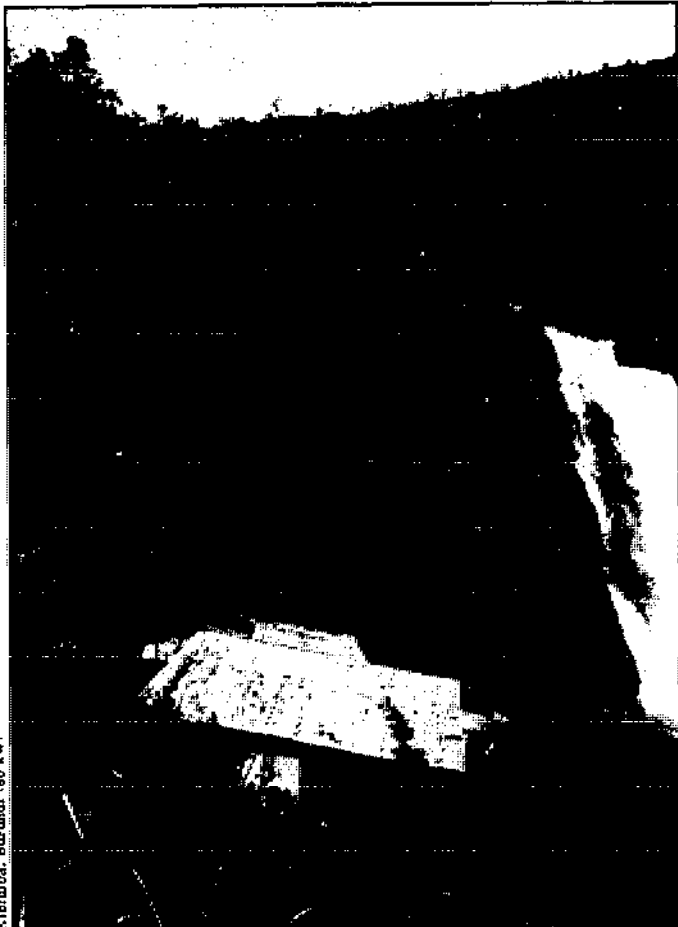
Fig. 5.166. Stones thrown on galvanized sheet roofing can pierce it. At this site, rainwater leaking through such a hole fell on the generator, causing a short and putting the plant out of commission until five years later when the rising price of diesel fuel forced the site owners to overhaul the generator.
