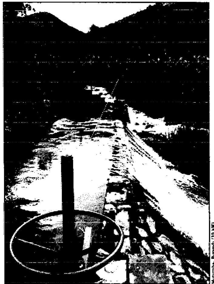
this area. Long spillways before and after the intake gate seen in the photograph on the right ensure a fairly constant level in the canal.
