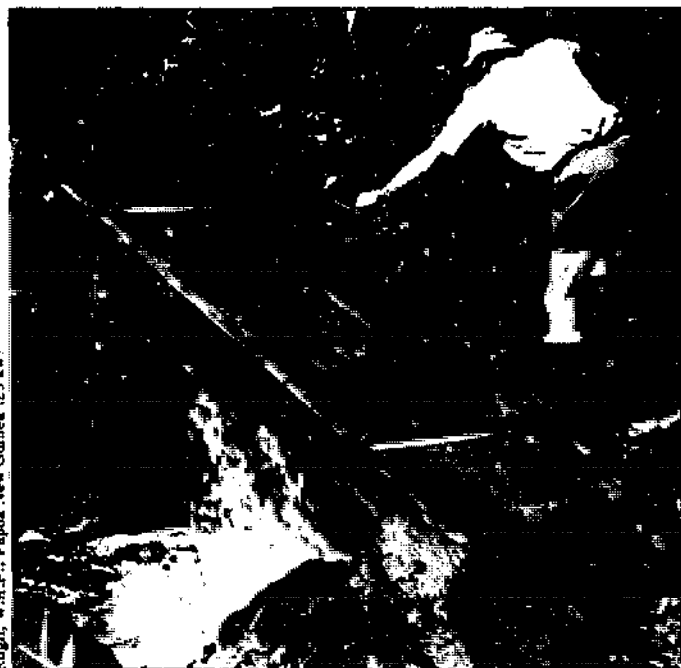
Fig. 5.99. A simple but effective gate in a sheet-metal flume.
