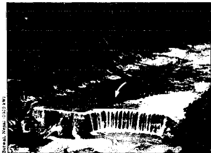
Fig. 5.28. A temporary diversion weir across the stream is used to divert water toward an underground intake at the left. This dam is used only to increase head; it does not form a reservoir to store water.
