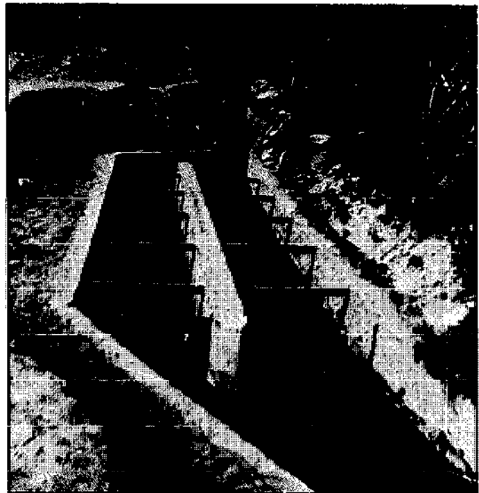
Fig. 5.199. This settling basin just after the intake incorporates two sections—one can be cleaned out while the other remains in use. No scouring outlet has been incorporated, and sediment has to be shoveled out.
