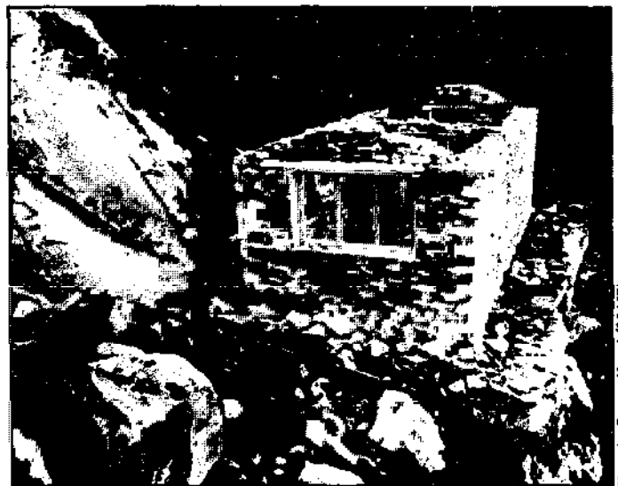
Fig. 5.161. A powerhouse constructed of dry-rubble masonry.
