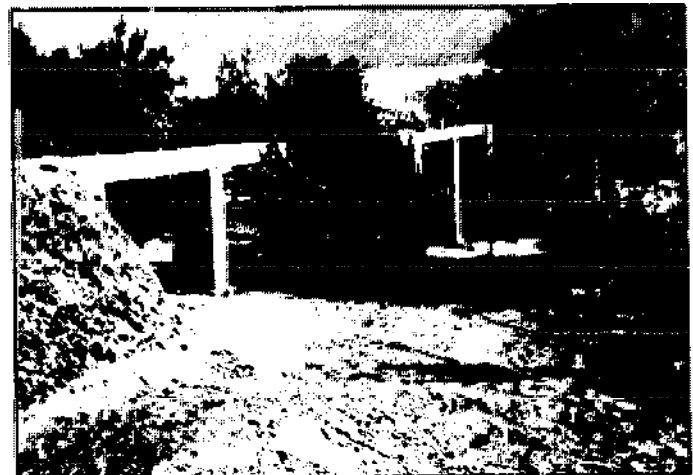
Fig. 10.49. A flume constructed of concrete and supported by masonry pillars conveys water from the canal to the powerhouse (behind the trees) at Bunjl.
