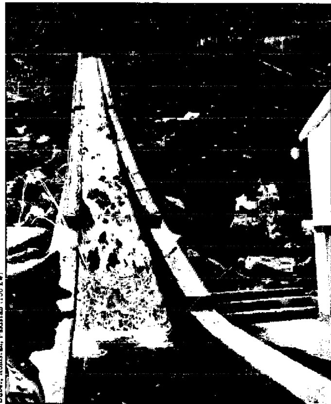
Fig. 5.16. Excess water is led around the powerhouse back into the tailrace canal. Stones embedded in the concrete chute dissipate the energy of the descending water.
