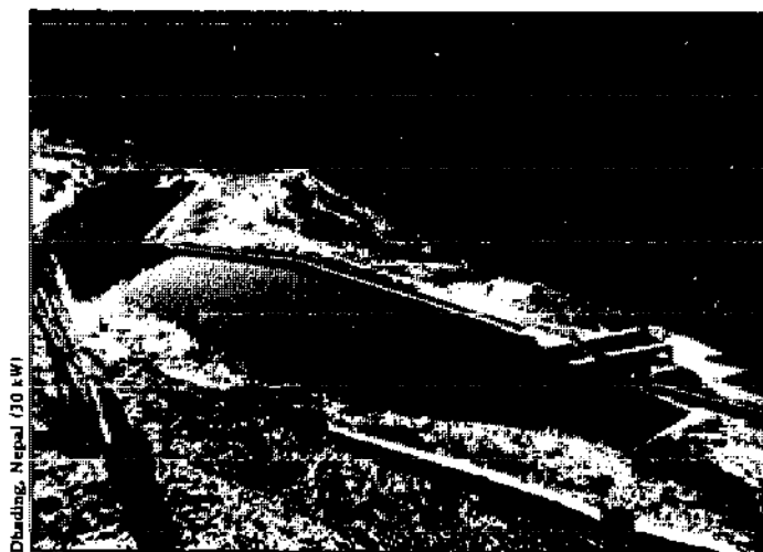
Fig 5.120. A forebay used to store water for power generation during peak demand periods.
