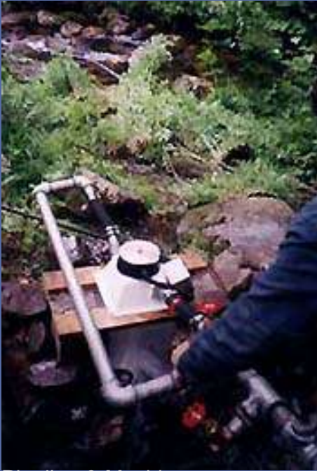
Pipeline & Machine (Photo by Jo Pach)
