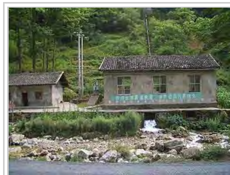
Hongping Power station, in Hongping Town, Shennongjia, has a design typical for small hydro stations in the western part of China's Hubei Province. Water comes from the mountain behind the station, through the black pipe seen in the photo
