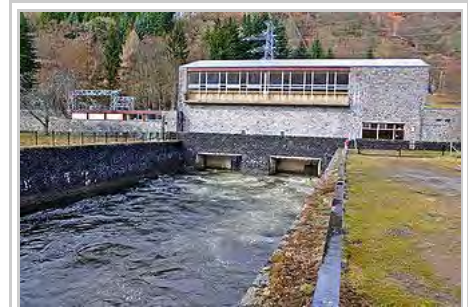
Small 2MW hydro in Perthshire, Scotland
