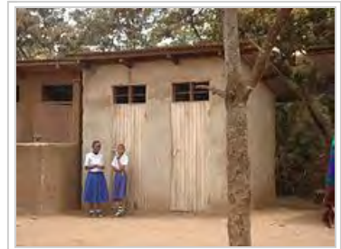
School toilets for girls in Tanzania, if they exist, often have no facilities to dispose of pads.
