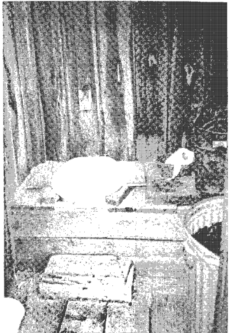
AN OUTDOOR SAWDUST TOILET BUILT OF RECYCLED MATERIALS. A REMOVABLE BUCKET LINGERS UNDER THE TOILET SEAT, WAITING TO BE FILLED, EMPTIED AND COMPOSTED.
