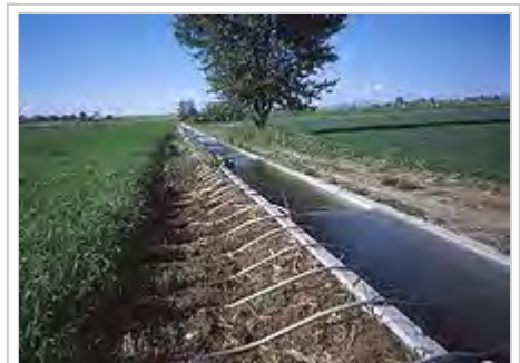
Furrow irrigation system using siphon tubes
