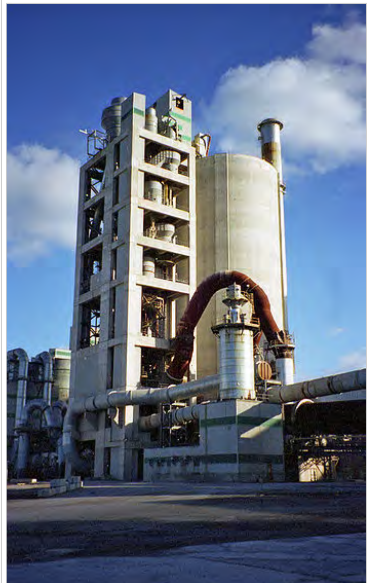
A preheater tower, rawmix silo and exhaust stack. Bottom left: rawmill. Bottom right: rotary kiln with tertiary air duct above. The U-shaped duct leading from the kiln inlet is an "alkali bleed".
