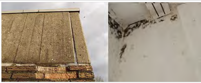
Moldy housecorner from outside and inside
