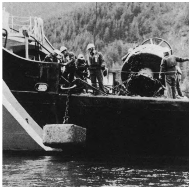
Figure 512. A sinker used to anchor a buoy.
