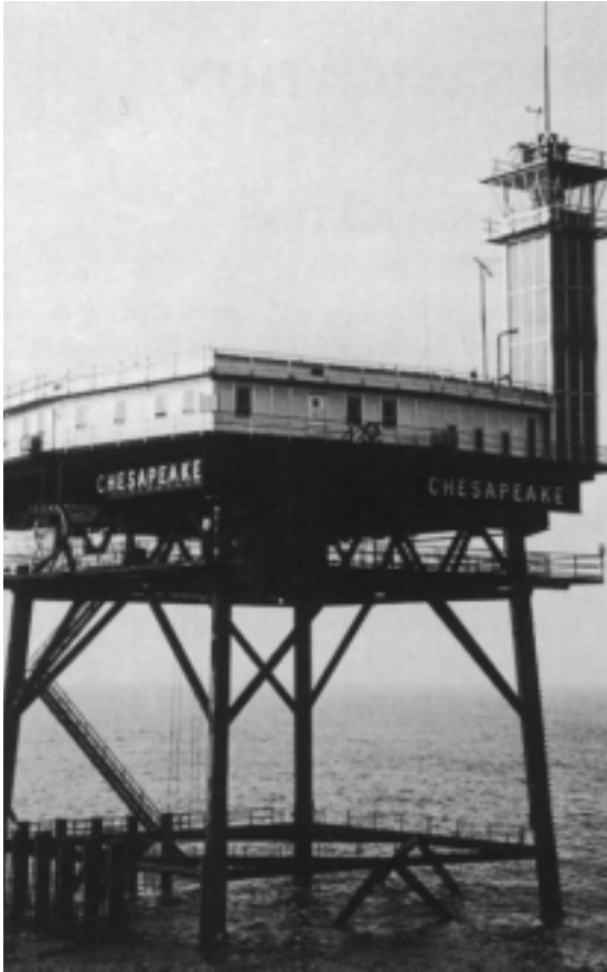
Figure 501a. Typical offshore light station.
