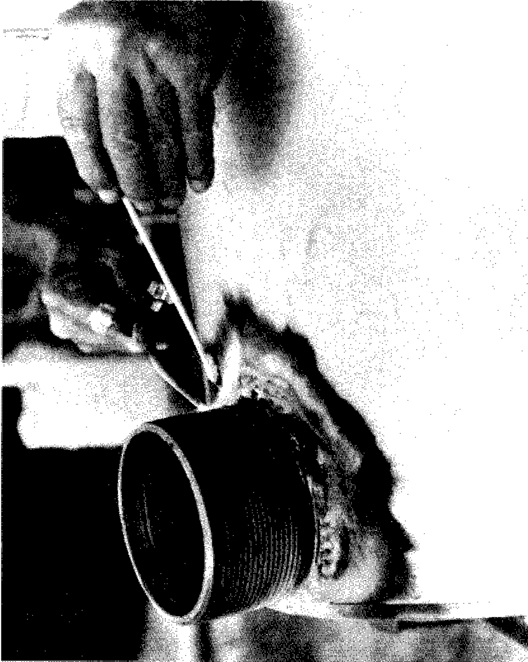
Fig. 2-7. Braze, do not weld , the plumbing fittings to the thin walled drums.
