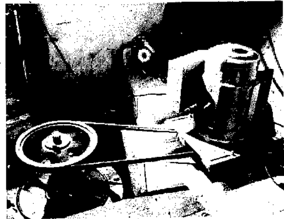
The Evans 6kW propeller turbine pilot installation (the belt guards are not yet fitted).
