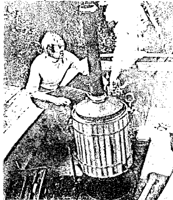
Vertical Coal Fired Boiler
