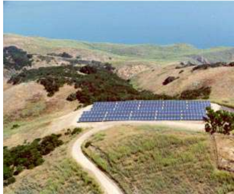
ETS staff managed this PV installation off the California coast on Santa Cruz Island. This 130 kW site validates the cost-effectiveness of renewable technologies in isolated, remote applications.
