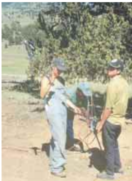
Leveling the tower and tensioning guy cables with a come-along.
