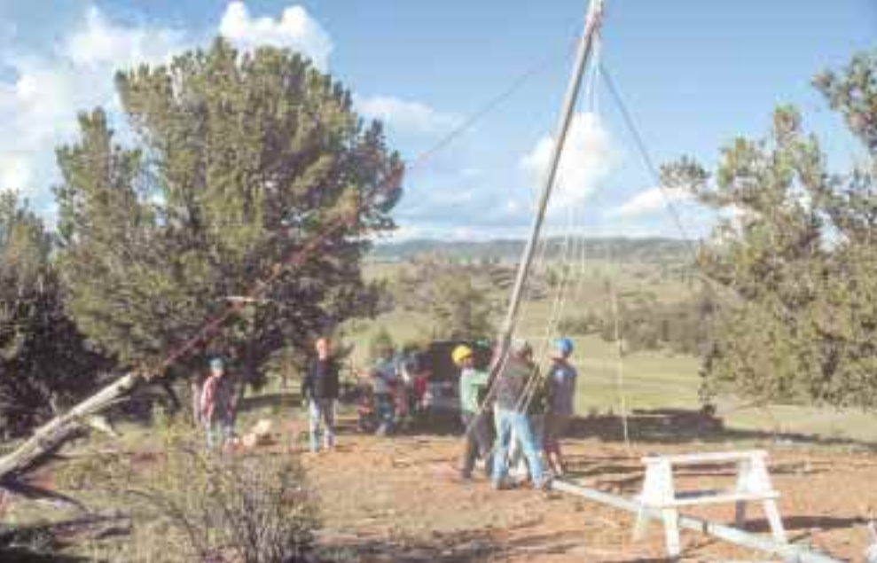
“Heave-ho”ing the tower gin pole into place.
