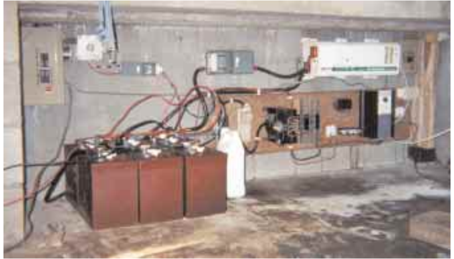
The Bosque del Cabo system utilizes a 1 1/2 HP motor (left) to produce 180 watts from 21 gpm at 190 feet of head. 2,300 feet from the hydro unit, the rest of the system (right) steps down from 415 VAC to 12 VDC.
