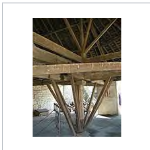
Main axle of mill. Roof truss above is separate; mill's own tie beam visible between.
