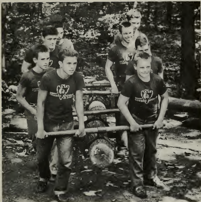
Moving Heavy Timber—Use of Log Carriers
