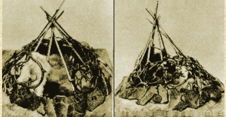
Circular tents from Malta, Siberia. These animal hide covered structures were bolstered with stones at the base.
