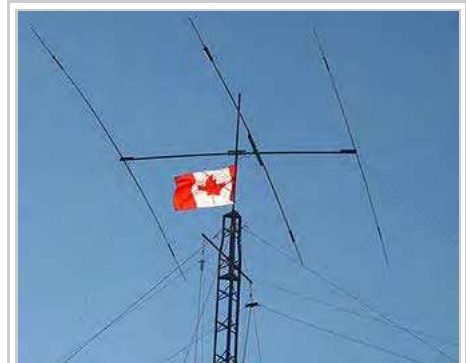
The top of a tower supporting a Yagi-Uda antenna and several wire antennas
