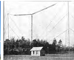
T antenna of amateur radio station, 80 ft high, used at 1.5 MHz.
