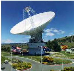
NASA Cassegrain parabolic spacecraft communication antenna, Australia. Uses X band, 8 – 12 GHz. Extremely high gain ~70 dBi.
