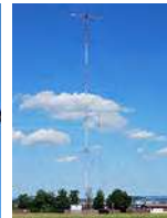
Mast radiator antenna of medium wave AM radio station, Germany
