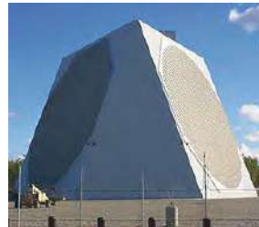
US Air Force PAVE PAWS phased array radar antenna for ballistic missile detection, Alaska. The two circular arrays are composed of thousands of crossed dipole antennas.
