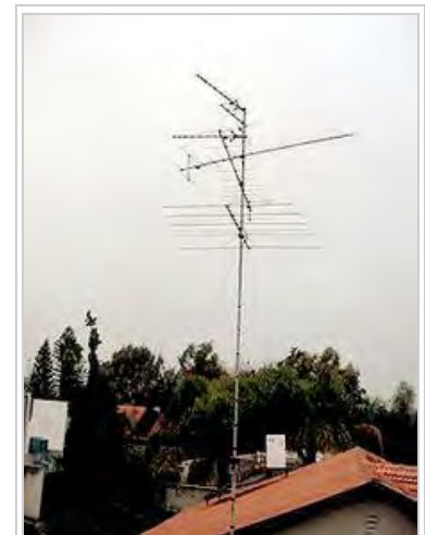
Rooftop television Yagi-Uda antennas like these are widely used at VHF and UHF frequencies.
