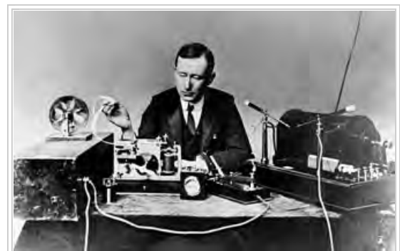
Guglielmo Marconi who built the first radio receivers, with his early spark transmitter ( right ) and coherer receiver ( left ) from the 1890s. The receiver records the Morse code on paper tape
