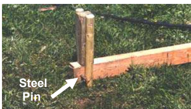
5f Streambank Arm Detail
