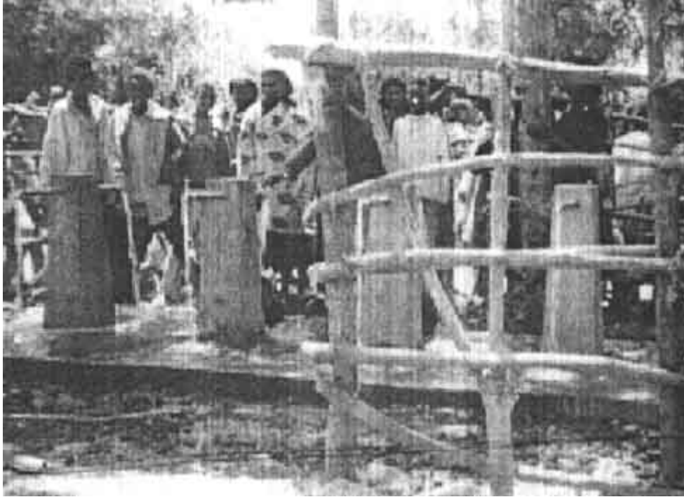
Fig.7 Water Supply System at Dodicha Woreda, Arsi Zone, Oromia Region from RDTAC's Hydram
