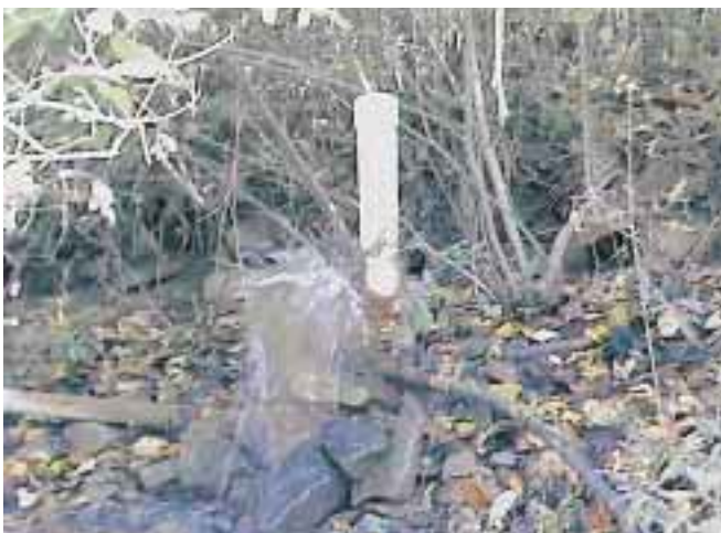
Scott Lee's ram pump in operation.
