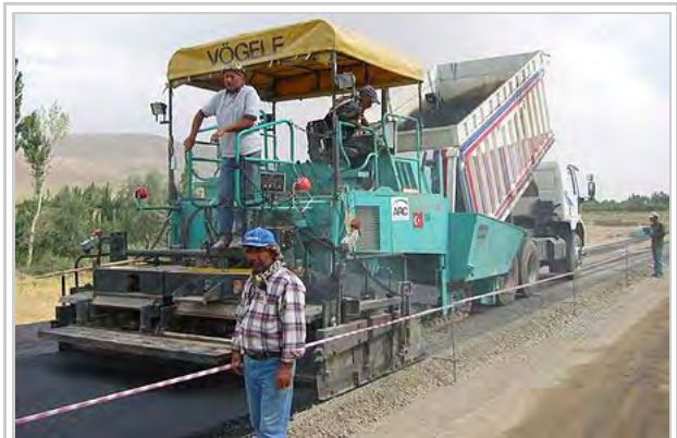
A machine laying asphalt concrete, fed from a dump truck
