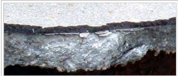
As shown in this cross-section, many older roadways are smoothed by applying a thin layer of asphalt concrete to the existing portland cement concrete, creating a composite pavement.
