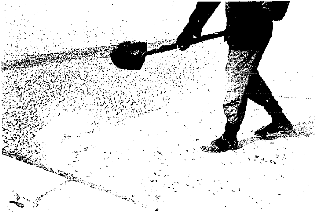
Figure 3. Spreading fine aggregate for dry-bound macadam
