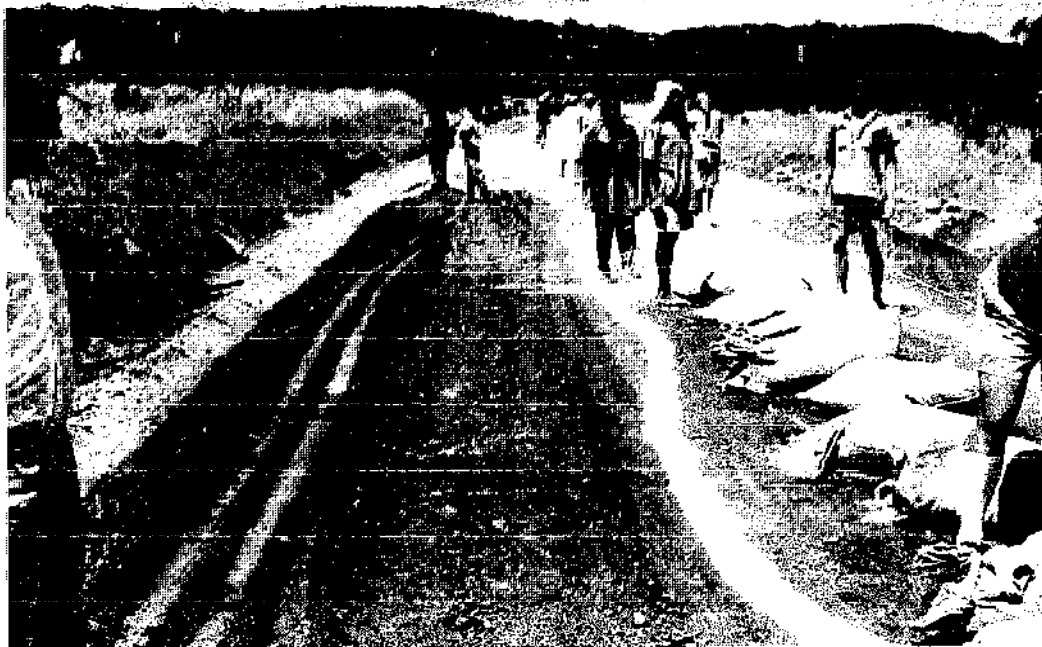
Figure 5. Lime stabilisation: bags of lime are dumped along the road
