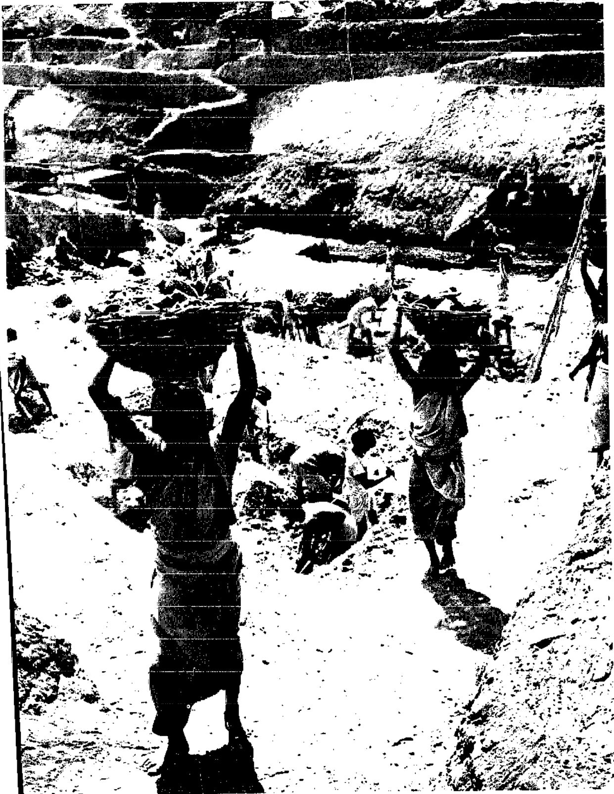
Figure 19. Use of head baskets to carry excavated material (India)
