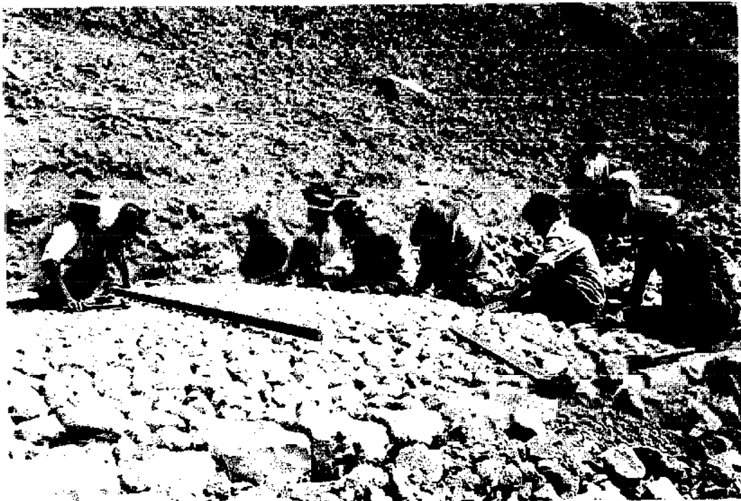
Figure 9. Cobblestone road construction
