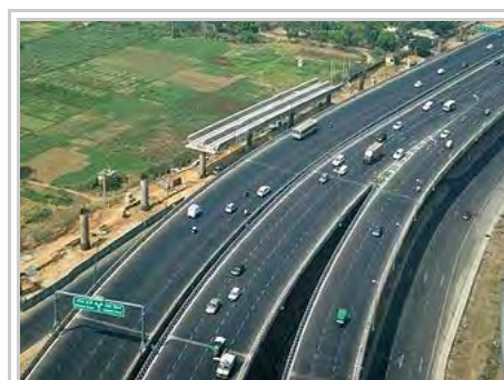
A dual carriageway section of National Highway 8 connecting Delhi to Gurgaon
