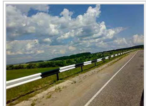
Road with guard rails in Kaluga Oblast, Russia
