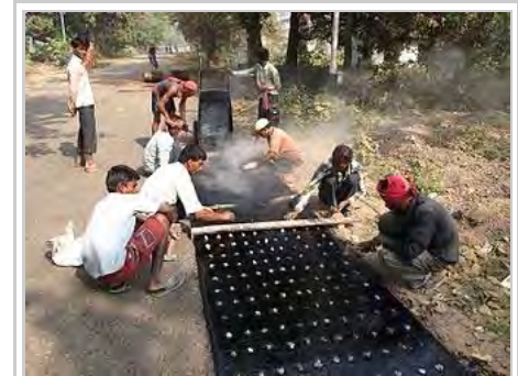
Manual road repair taking place in Howrah, India
