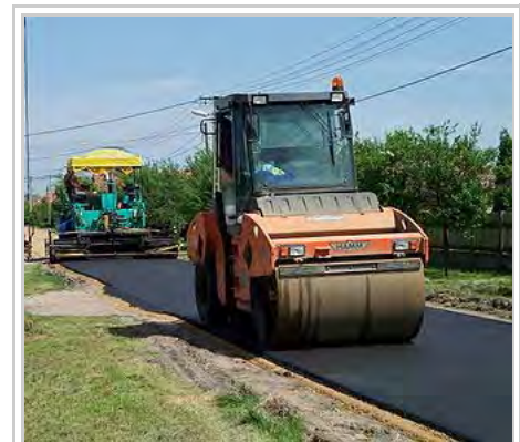
Asphalt layer and Hamm road roller
