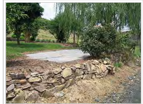
Septic tank in Lesotho (underground), concrete cover slab is visible
