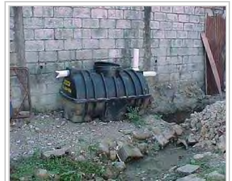
A septic tank before installation, with manhole cover on top
