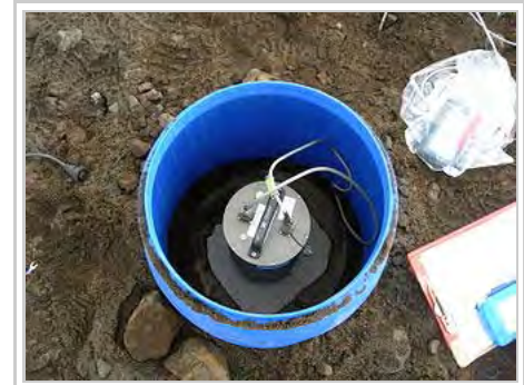
Installation for a temporary seismic station, north Iceland highland.
