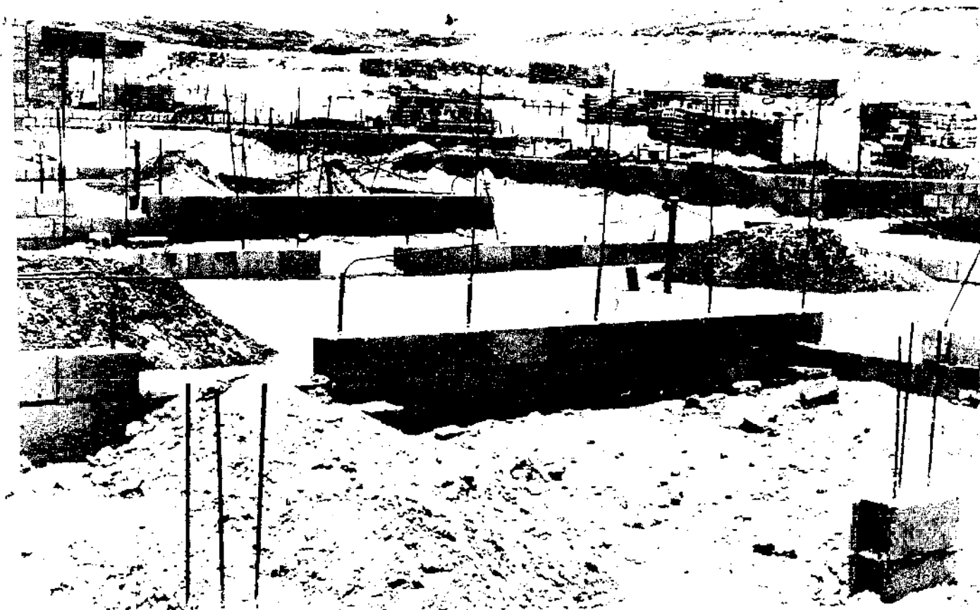
FIGURE 24 REINFORCED CONCRETE MASONRY WALLS UNDER CONSTRUCTION FOR HOUSING IN CENTRAL LUZON, THE PHILIPPINES.
