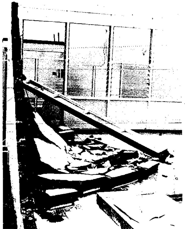
FIGURE 12 SINGLE FAMILY HOUSE SHOWING COLLAPSE OF ROOF AND EXTERIOR WALL DURING THE PHILIPPINES TYPHOON IN NOVEMBER 1970.
