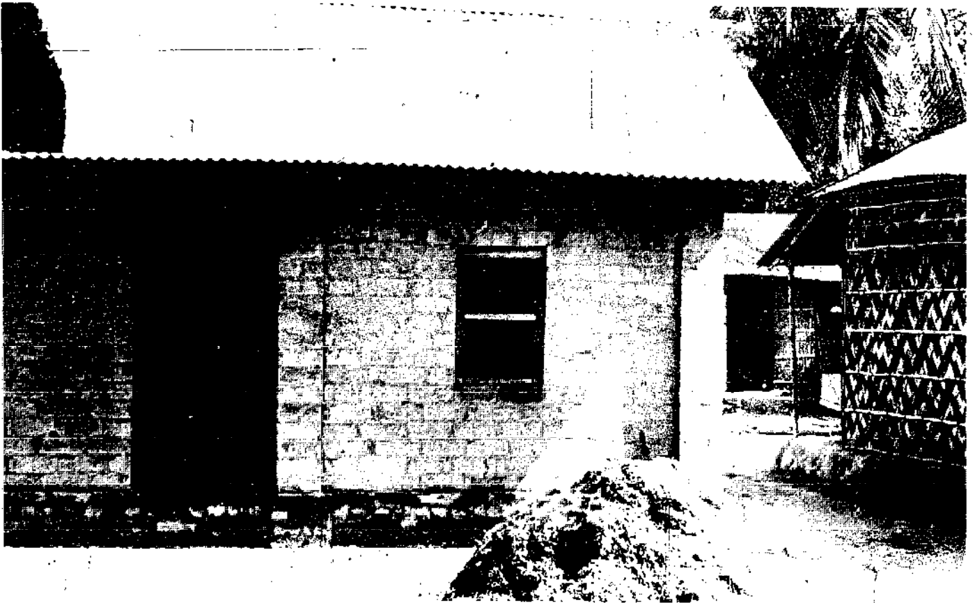
FIGURE 27 CARE SPONSORED HOUSING PROJECT NEAR DACCA, BANGALADESH SHOWING CINVA-RAM WALL CONSTRUCTION WITH CORRUGATED METAL ROOFING.
