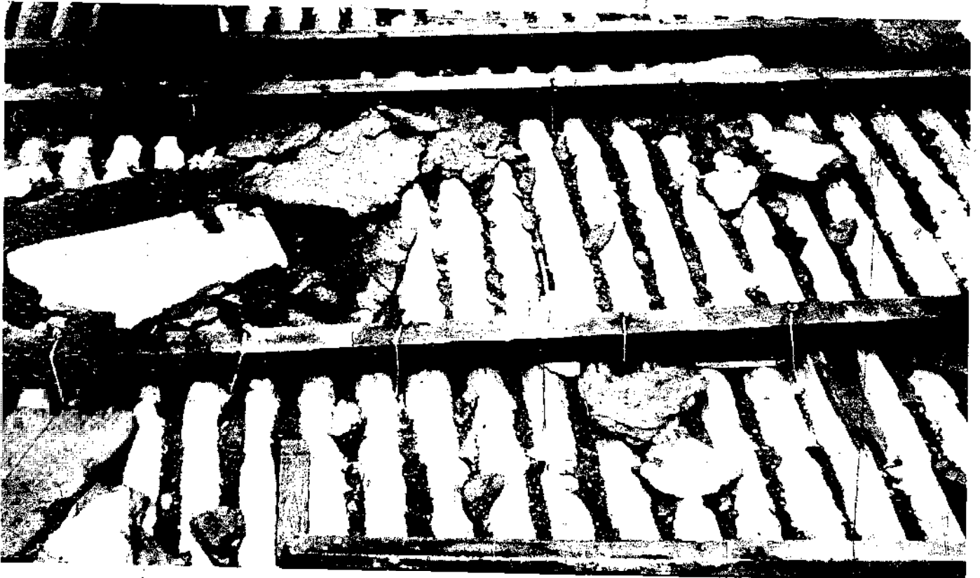
FIGURE 50 ALTHOUGH THE ROOF BLEW OFF OF THE STRUCTURE, THE CORRUGATED ROOFING WAS EFFECTIVELY TIED TO PURLINS BY WIRES COMPLETELY AROUND THE PURLINS.
