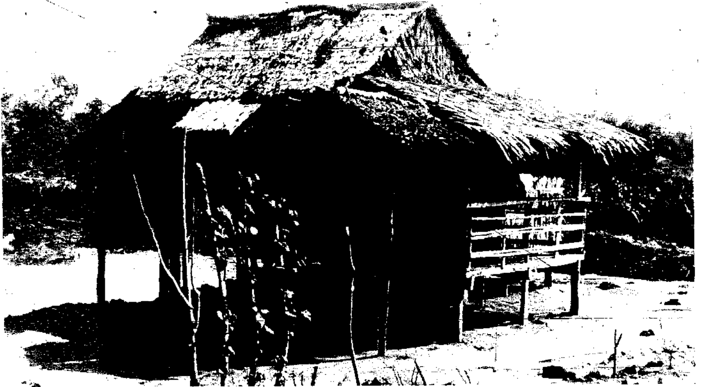
FIGURE 39 POLE-TYPE CONSTRUCTION.
