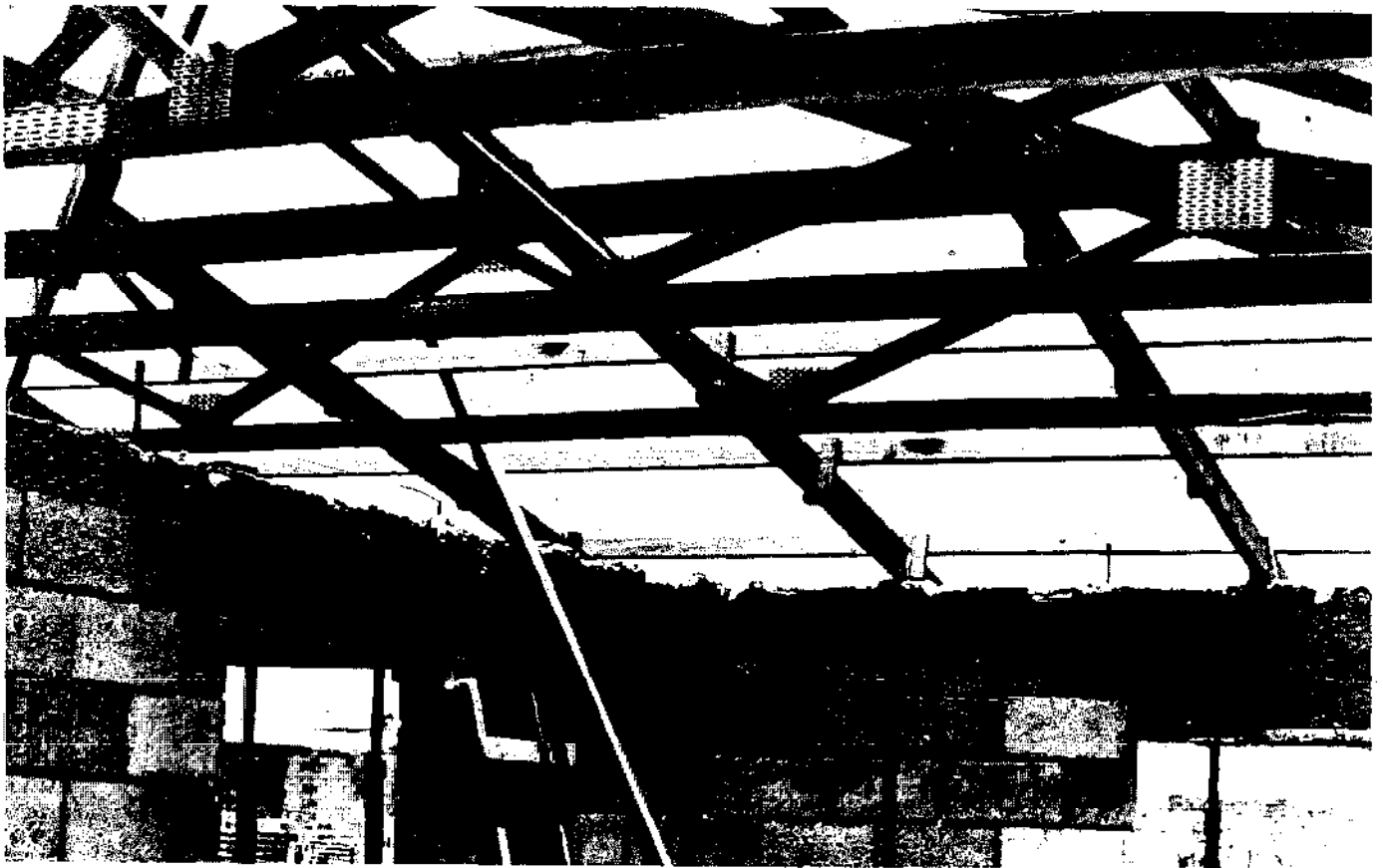
FIGURE 25 CONCRETE MASONRY BEARING WALL CONSTRUCTION WITH TRUSS TYPE ROOF FOR HOUSING IN CENTRAL LUZON, THE PHILIPPINES.
