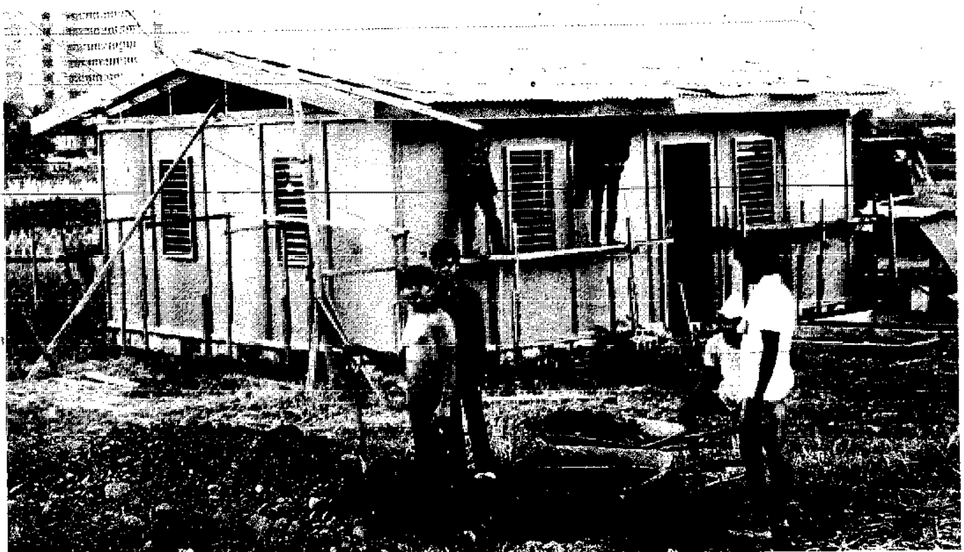
FIGURE 40 WOOD-FRAME WALL AND ROOF.
