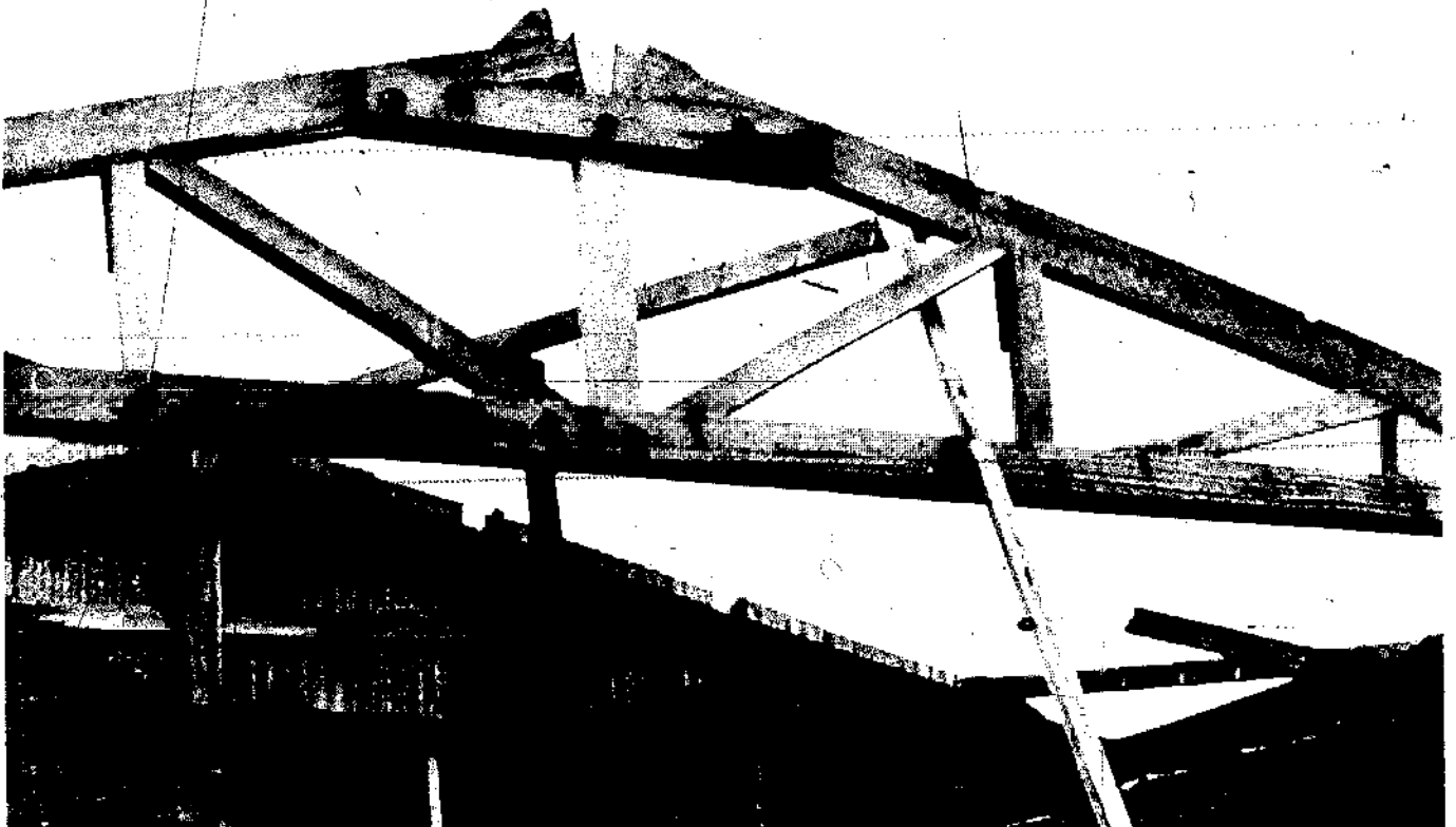
FIGURE 10 ROOF FAILURE IN BUILDING CAUSED BY NOVEMBER 1974 TYPHOON IN THE PHILIPPINES.
