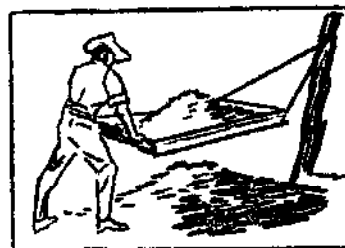
Fig. 6 - Screening the Soil
