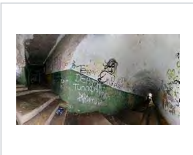
Inside the Hill 60 Bunker, Port Kembla, New South Wales. One of many bunkers south of Sydney
