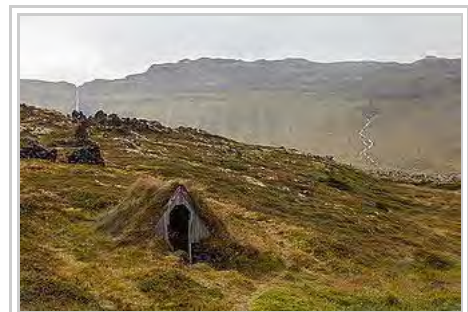
Example of an abandoned Icelandic turf house in the region of Búðahreun via earth berming
