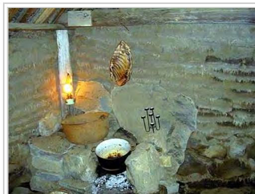
Turf house in Sænautasel, Iceland. Inside view showing the turf layers on the walls.
